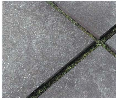
Installation onto grass
