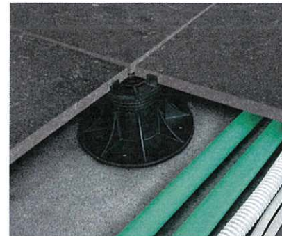
Raised installation onto support structures
