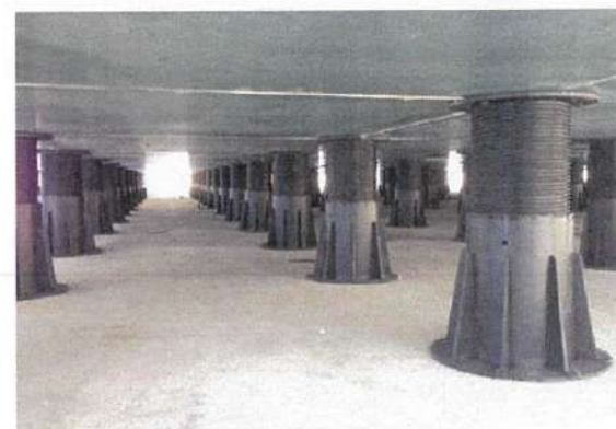
Project in Chile (Pedestal Paving)
